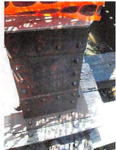
60-NCRR Ped Bridge_Y14_L8 North End
