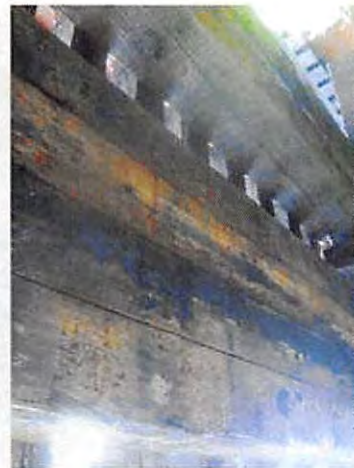
108-NCRR Ped Bridge_Y14_Timber bottom
