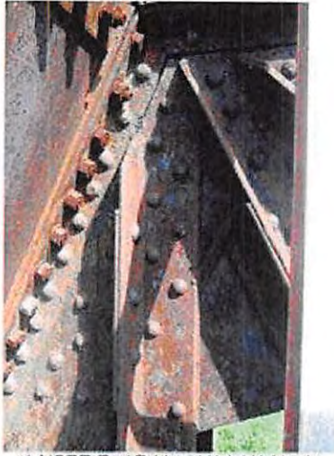
1-NCRR Ped Bridge_Y14_U1 North
