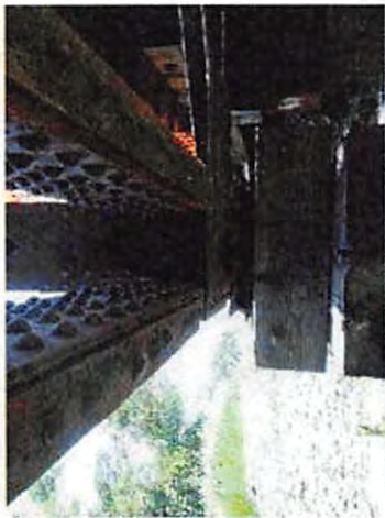
85-NCRR Ped Bridge_Y14_L0 South interior
