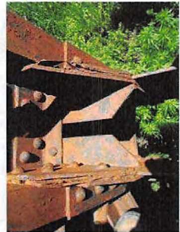
63-NCRR Ped Bridge_Y14_L1 South west.
