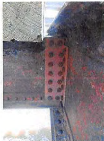
44-NCRR Ped Bridge_Y14_Bay 4 Stringer 1 Newer clip angle
