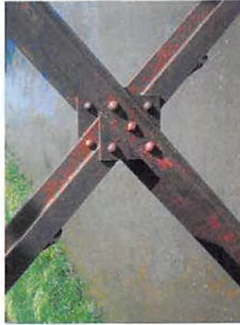
119-NCRR Ped Bridge_Y14_Diagonal connection
