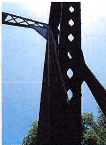
71-NCRR Ped Bridge_Y14_U7L7 South Interior bent
