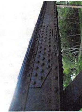
26-NCRR Ped Bridge_Y14_U2U3 South Splice
