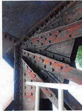
17-NCRR Ped Bridge_Y14_U7 North
