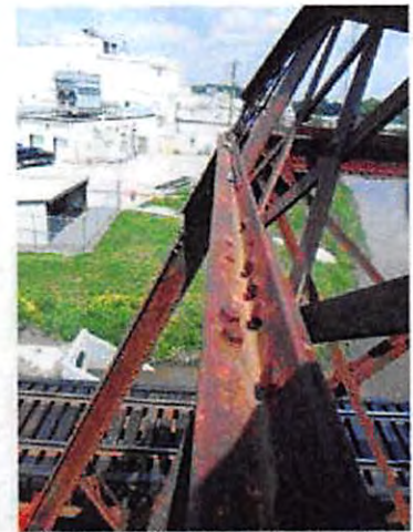
36-NCRR Ped Bridge_Y14_West portal bracing
