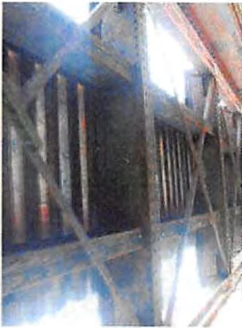
103-NCRR Ped Bridge_Y14_Typ. truss bay
