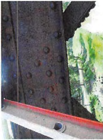
22-NCRR Ped Bridge_Y14_U5 South
