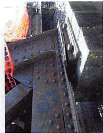
90-NCRR Ped Bridge_Y14_L0 North
