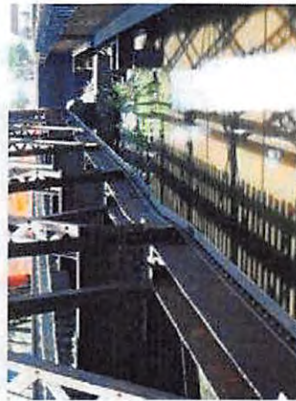
56-NCRR Ped Bridge_Y14_North Truss lower chords looking west
