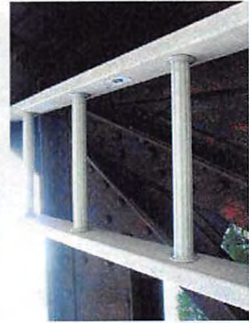
33-NCRR Ped Bridge_Y14_U1 South
