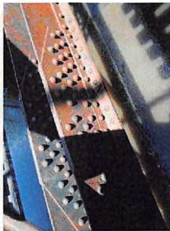
50-NCRR Ped Bridge_Y14_L5L6 North splice
