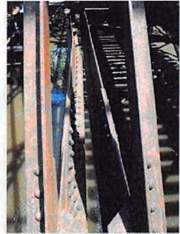
48-NCRR Ped Bridge_Y14_U5L6 North bent exterior
