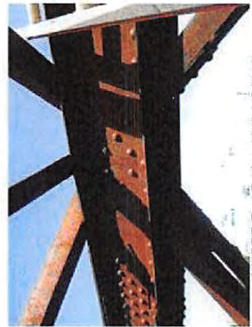
6-NCRR Ped Bridge_Y14_U3 North
