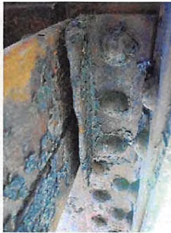
104-NCRR Ped Bridge_Y14_Bent stringer seat
