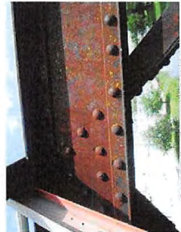
9-NCRR Ped Bridge_Y14_U4 North
