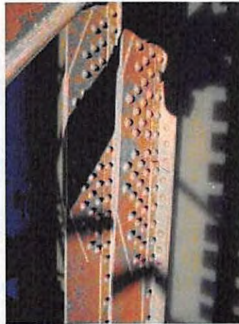
41-NCRR Ped Bridge_Y14_L2L3 North Splice
