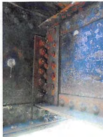
86-NCRR Ped Bridge_Y14_Typ. Stringer clip angle
