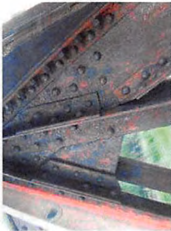
31-NCRR Ped Bridge_Y14_U1 South
