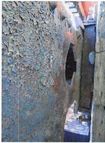
91-NCRRR Ped Bridge_Y14_L0 North interior
