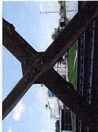
47-NCRR Ped Bridge_Y14_U2L4 North interior bent at U5L3 North connection
