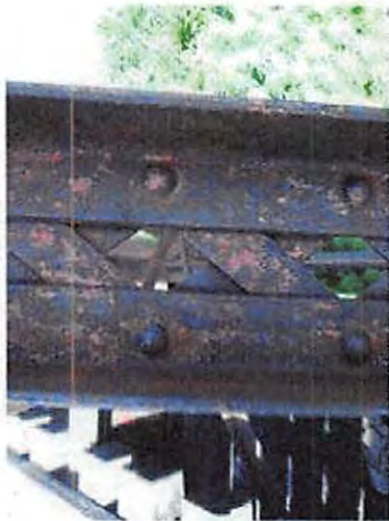
97-NCRRR Ped Bridge_Y14_Typ_First diagonal
