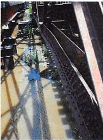
49-NCRR Ped Bridge_Y14_L5L6 North bent exterior
