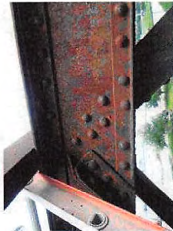
16-NCRR Ped Bridge_Y14_U6 North
