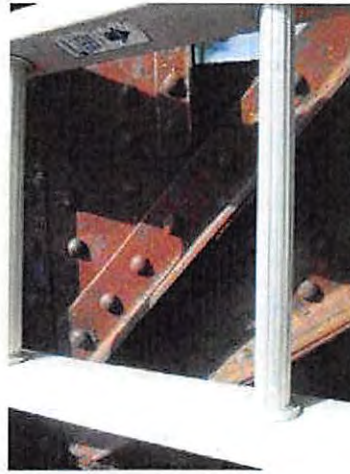
2-NCRR Ped Bridge_Y14_U1 North
