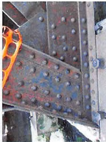
59-NCRR Ped Bridge_Y14_L8 North Exterior
