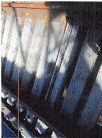
115-NCRR Ped Bridge_Y14_Heavy tie...
