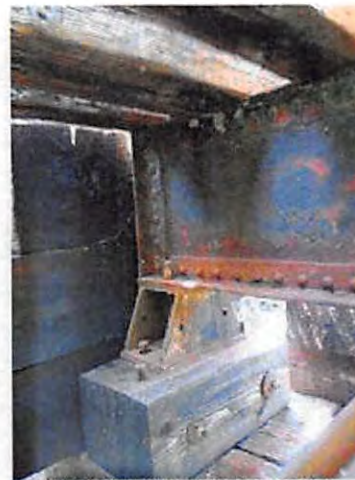
89-NCRR Ped Bridge_Y14_Typ. Stringer at end
