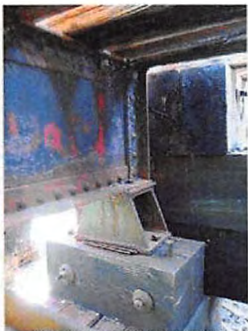
88-NCRR Ped Bridge_Y14_Typ. Stringer at end
