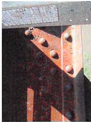
5-NCRR Ped Bridge_Y14_U2 North
