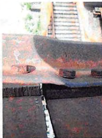
35-NCRR Ped Bridge_Y14_Southwest Portal bracing bent connection
