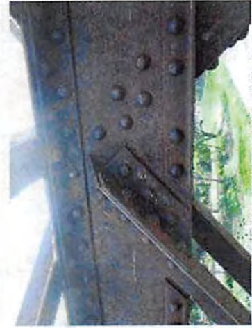
30-NCRR Ped Bridge_Y14_U2 South
