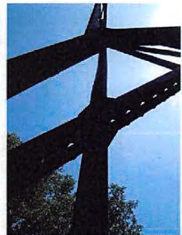
72-NCRR Ped Bridge_Y14_U7L7 South Interior bent
