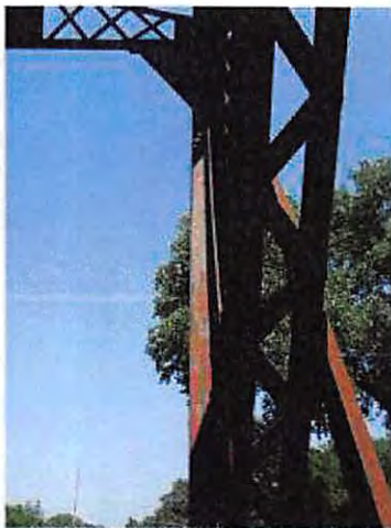
70-NCRR Ped Bridge_Y14_U7L6 South interior bent
