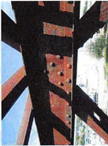
13-NCRR Ped Bridge_Y14_U5 North
