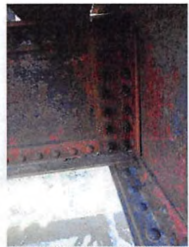
54-NCRR Ped Bridge_Y14_Bay 8 Str. 1 newer clip angle
