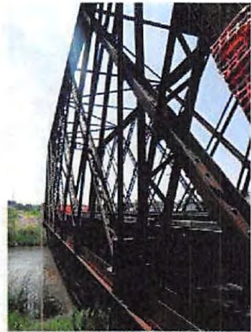
76-NCRRR Ped Bridge_Y14_South Truss Looking west
