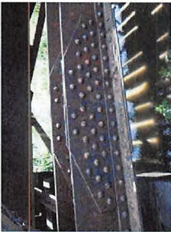
58-NCRR Ped Bridge_Y14_L7L8 North Splice
