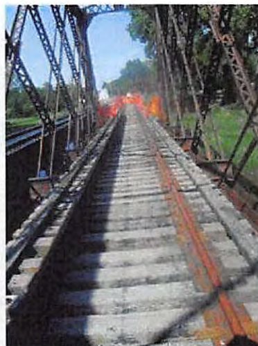
116-NCRR Ped Bridge_Y14_Deck ties
