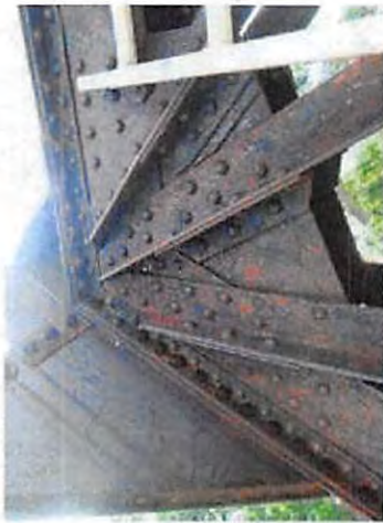
19-NCRR Ped Bridge_Y14_U7 South
