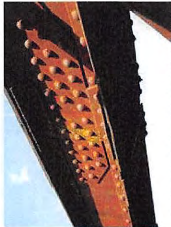
8-NCRR Ped Bridge_Y14_U2U3 North Splice
