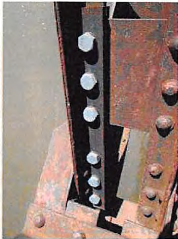
67-NCRR Ped Bridge_Y14_U3L5 South splice...
