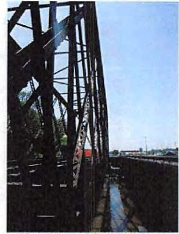
57-NCRR Ped Bridge_Y14_North Truss looking west
