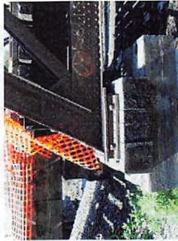
83-NCRR Ped Bridge_Y14_L0 South exterior
