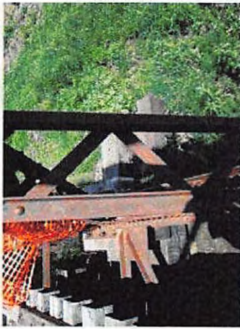
100-NCRR Ped Bridge_Y14_Typ. Truss diagonal
