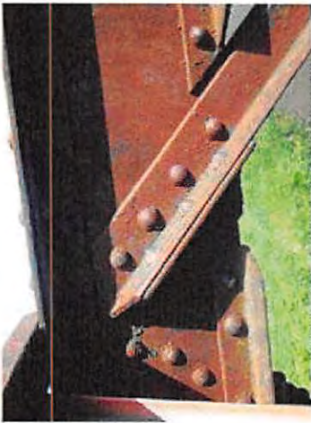
4-NCRR Ped Bridge_Y14_U2 North
