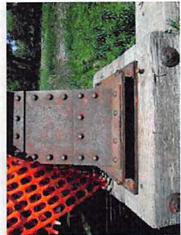
84-NCRR Ped Bridge_Y14_L0 South End
