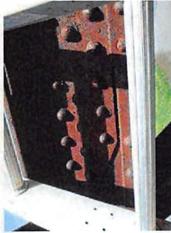
14-NCRR Ped Bridge_Y14_U5U6 North Splice
