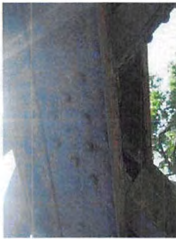
25-NCRR Ped Bridge_Y14_U4 South
