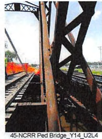
45-NCRR Ped Bridge_Y14_U2L4 North interior bent at U5L3 North connection
