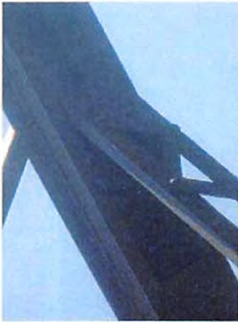
118-NCRR Ped Bridge_Y14_Upper
