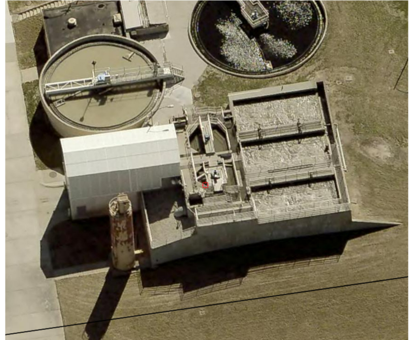
Existing Grit Removal Facility
