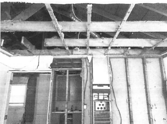
Fire Damaged Ceiling Removed
