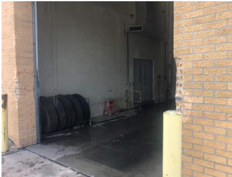
Figure 31. Damage to Brick Veneer (photo taken 6/25/19)
