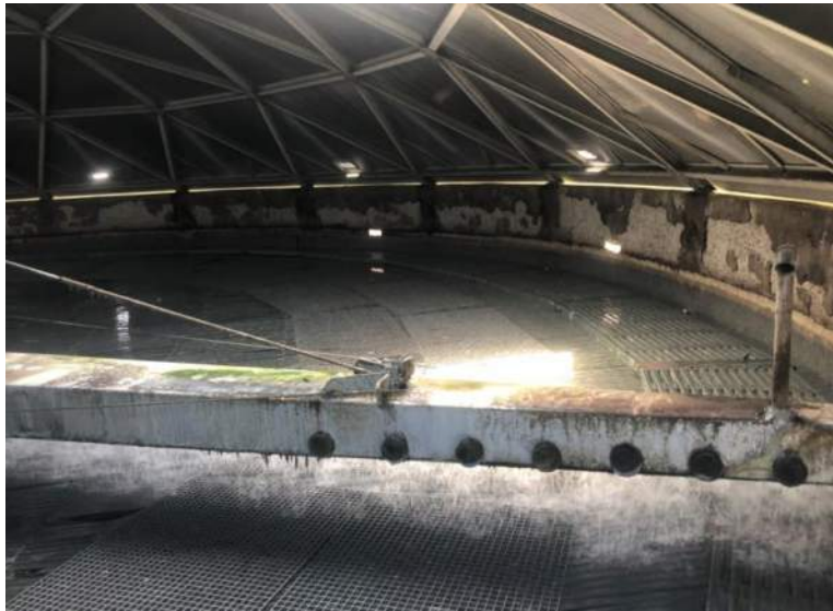
Figure 28. Inside Trickling Filter #1 (South) (photo taken 6/25/19)
