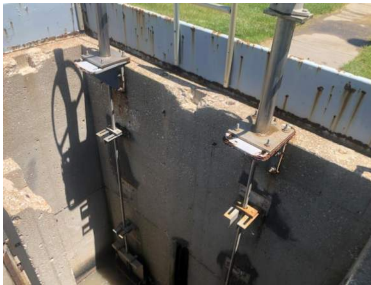
Figure 21. Existing Slide Gates (photo taken 6/25/19)
