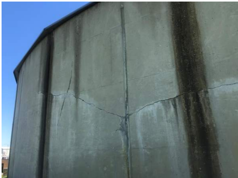
Figure 27. Cracking Observed on Trickling Filter #1 (South) (photo taken 6/25/19)
