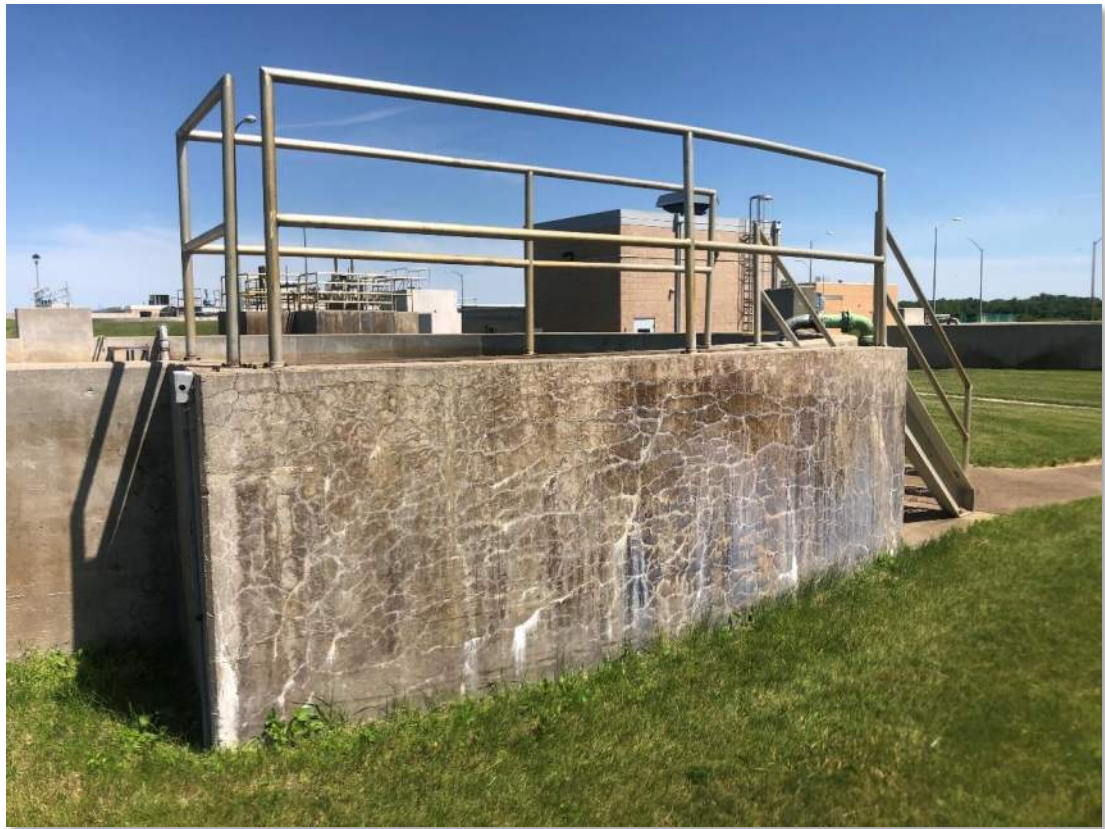
Figure 12. Photo of Aeration Basin #2 and Evidence of Alkali-Silica Reaction (ASR) Degradation
