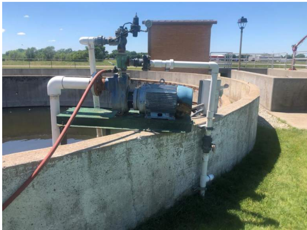
Figure 18. Photo of Irrigation Pump for WPC Site Irrigation (photo taken 6/25/19)
