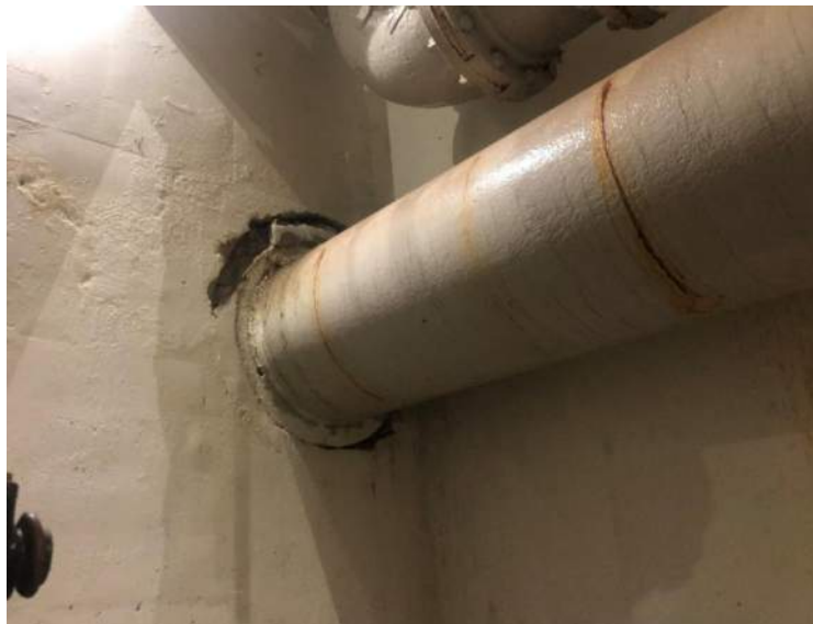
Figure 24. Failing Wall Connection (photo taken 6/25/19)
