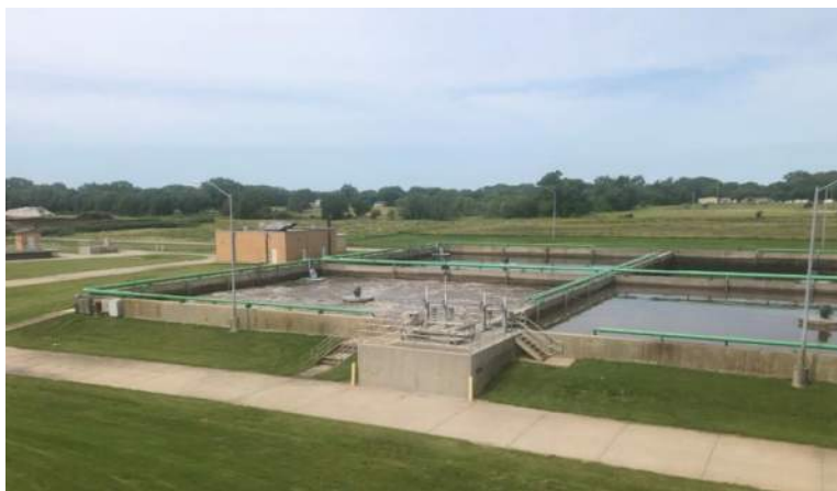
Figure 30. Existing Four-cell Sequencing Batch Reactor (SBR) Unit (photo taken 6/25/19)
