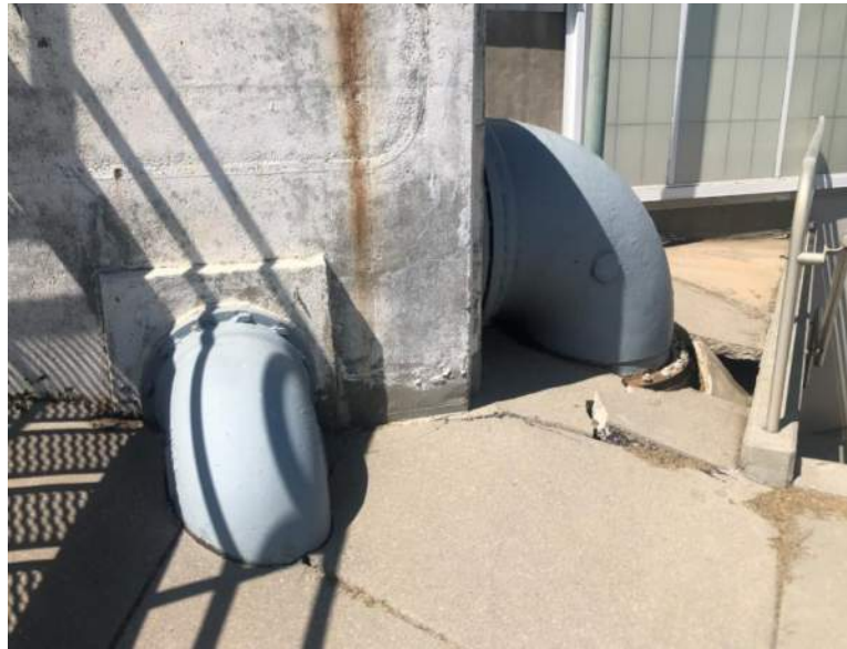
Figure 26. Concrete Upheaval at South Inlet Pipe (photo taken 6/25/19)
