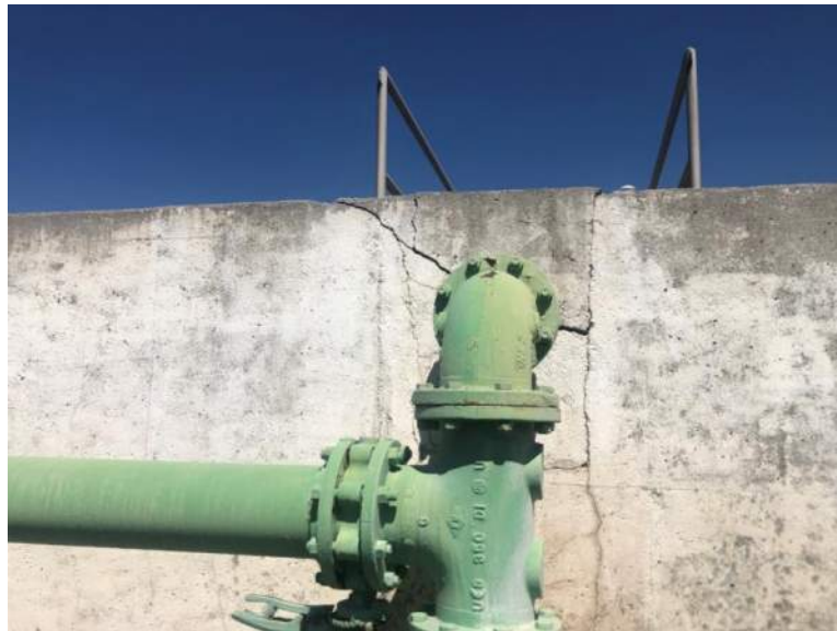
Figure 25. Concrete Cracking (photo taken 6/25/19)
