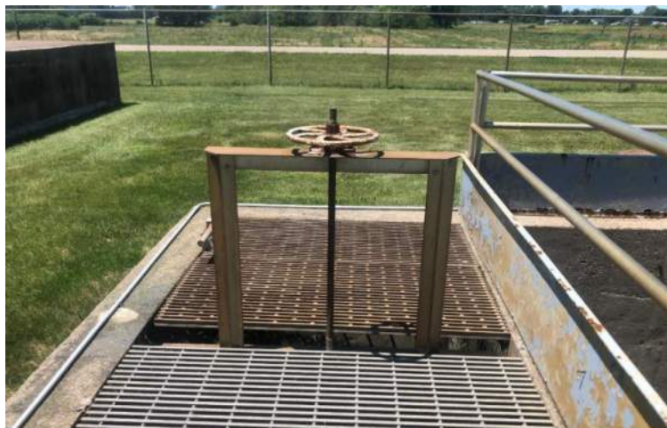
Figure 22. Abandoned Slide Gate (photo taken 6/25/19)
