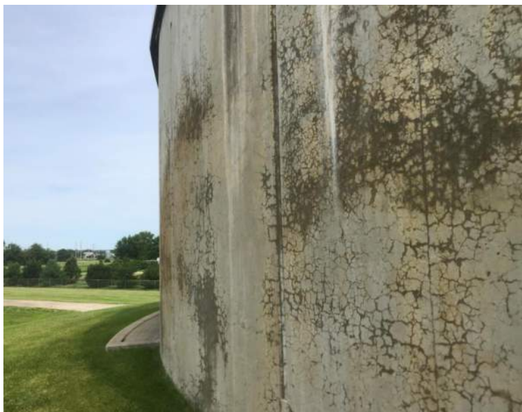
Figure 29. Alkali-Silica Reaction (ASR) of Trickling Filter #2 (North) (photo taken 6/25/19)
