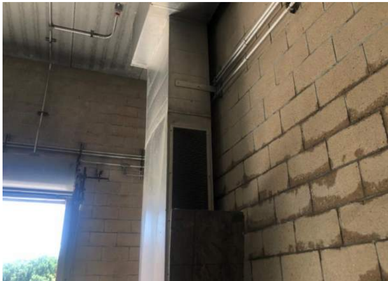
Figure 23. Moisture Seepage Through Concrete Masonry Unit Walls (photo taken 6/25/19)
